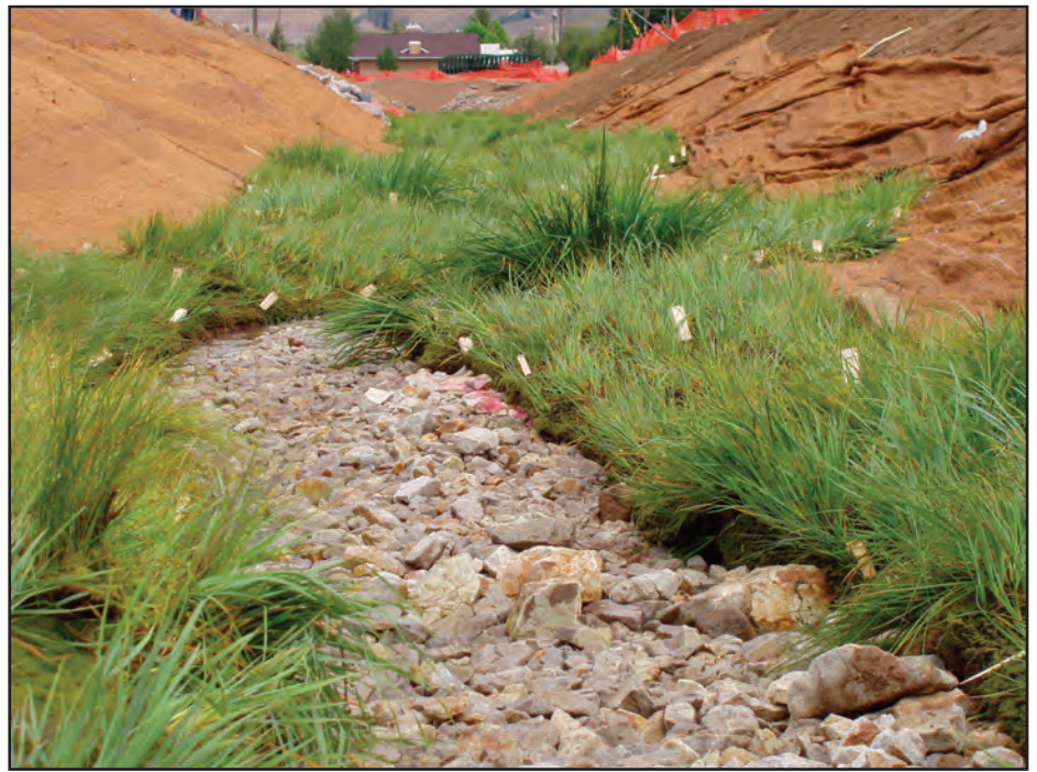
Prevegetated coir immediately after installation. Cover of native sedges and rushes is already quite dense, though not complete, and plants are primed for vigorous root growth.
