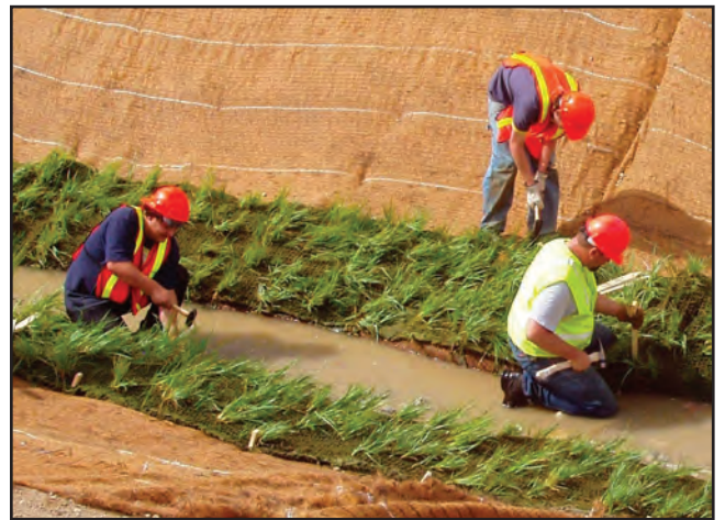
Butte-Silver Bow County crews stake prevegetated coir in place in August, 2004.
