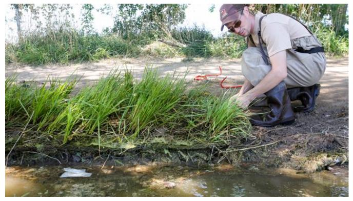
The wetland sod is made of a mixture of wooly sedge, beak sedge and arctic rush. The grasses are planted in short, rectangular patches along the shore but will grow to be around three feet tall and extend up the bank and into the water.
